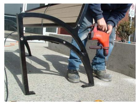
5. Put a 3 1/2" long, 3/8" diameter galvanized or stainless carriage bolt with washer through all the leg mounts. (Cascades Park series benches and picnic tables require a minimum of 8" bolts.)
