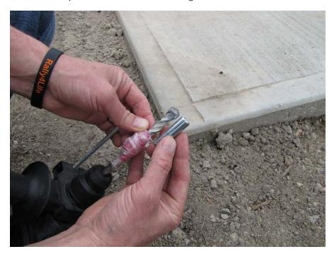
5. Drill the holes to a depth of 1-5/8" (as suggested by the anchor manufacturer).
