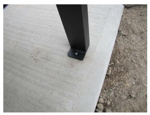
10. Secure bench to the anchor with bolt supplied.
