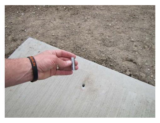
8. Hammer the anchor with the supplied post to expand the base securing it to the concrete.
