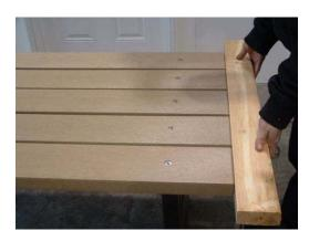
8. Secure nuts and washers to the bolts. DO NOT OVER TIGHTEN. The boards need to be able to expand and contract with changes in temperature.
