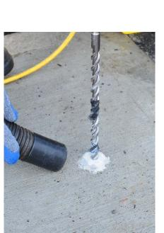
6. Insert concrete anchor. Use a spare bolt. Screw in a few turns and hammer down into the hole.
