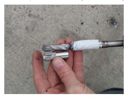
4. Drill the holes to the depth required – ensure drill is straight, perpendicular to ground.
