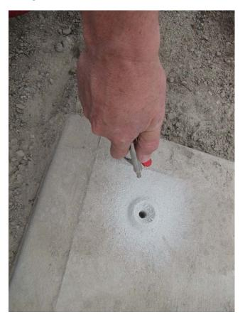
6. Insert concrete anchor - hammer the anchor with the supplied post to expand the base securing it to the concrete.
